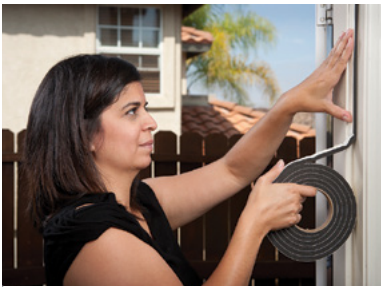
Installing weather stripping as part of SDG&E's Energy Savings Assistance Program
