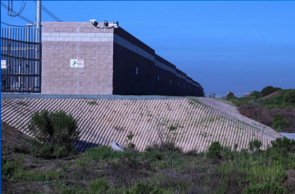
SDG&E's Bay Boulevard substation was built on a platform to raise it farther above sea level.
