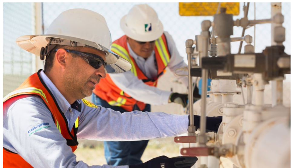
Our utilities work to protect system reliability.
